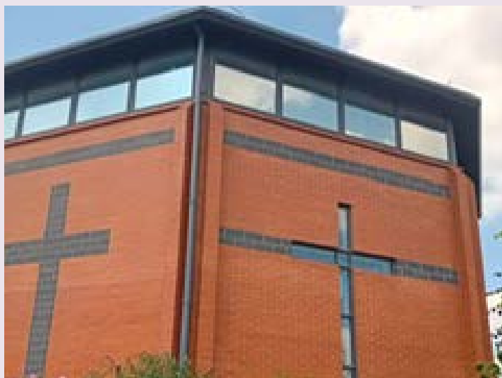
Outside South Norwood Baptist Church
